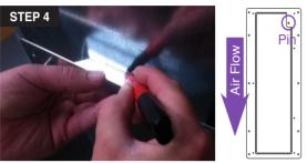
4. Screw the frame to the duct using the 12 provided self-tapping screws.
