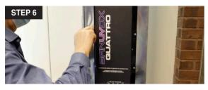
6. Unscrew the 6 retaining nuts and carefully **remove the unit from its mounting frame**.
