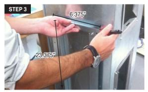
3. Use the frame as a template to cut a rectangular hole in the duct where the unit will be installed. The duct opening window should have the following dimensions: approximately 23.375" x 6.375".
