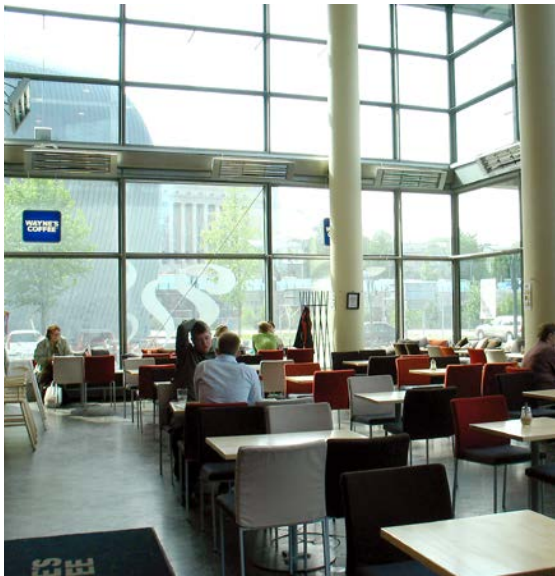
The IR heater can be mounted in an angled position to direct the heating where it is needed. Heaters used outdoors should be placed under a roof.
