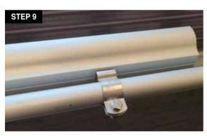
The IL Coil Clean assembly must be installed with the UV lamp facing the coil. Rotate the assembly into position and then tighten the setting screws on each of the mounting flanges.
