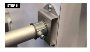
Once the assembly (rod and flanges) is positioned, secure the flanges to the walls of the HVAC unit using self-tapping screws. Be sure to level the assembly.
