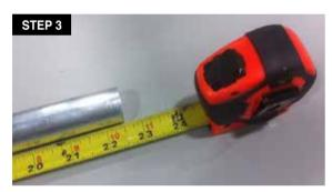
3. **Measure and cut the rod to desired length** or assemble several rods using couplers, if necessary.
