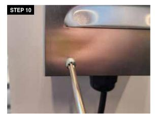
10. **Installation of the ballast box:** Remove the Phillips screws (4) from the ballast box cover. Set aside the bag containing the Gaynor plug and lamp boot. Mount the ballast box outside the air handler, on a wall or other hard surface. Screw it through the 2 holes in the center of the ballast box.
