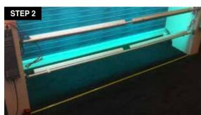
2. Locate the propre place where the installation will take place and measure the distance from one partition to the other: subtract 1.5" to take into account the two mounting flanges.
