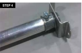
4. Place the mounting flanges on both ends of the support rod and insert this assembly into the HVAC unit at the desired height and depth.
