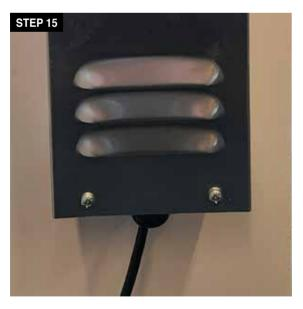
15. There remains only the **connection of the power supply** which **must be carried out by a certified electrician:** With the ballast box cover removed, install a connector on the round knockout on the bottom of the ballast box. Next, pull an appropriate power cable into the box. Insert the white (neutral) wire and the black (live) wire into the yellow quick connect module.
