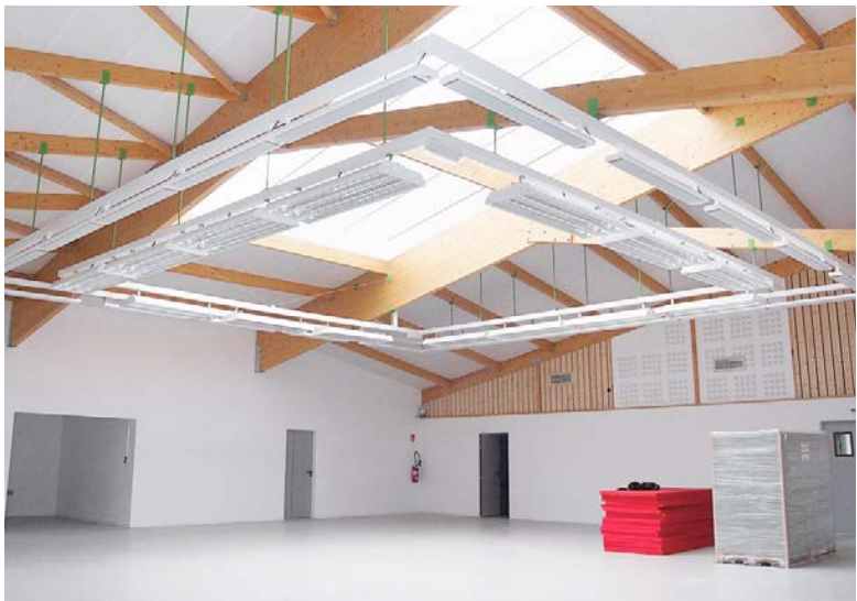
Buildings that are used on an irregular basis can be heated fast without a high energy consumption. EZ100 blends well with electrical fittings.
