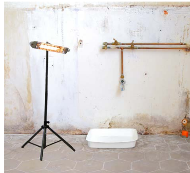
With its concentrated heat ELIR is a good complement to dehumidifiers for drying in areas damaged by water.
