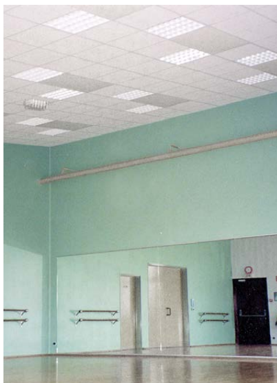
Thermocassette creates a pleasant heat on the floor in premises where you might want to be barefooted.
