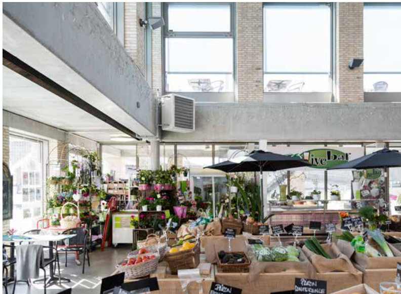
By turning the SWH, pipe connections are possible on both sides which makes it very easy to position. The air director, which has individually adjustable louvres directs the air flow as required.
