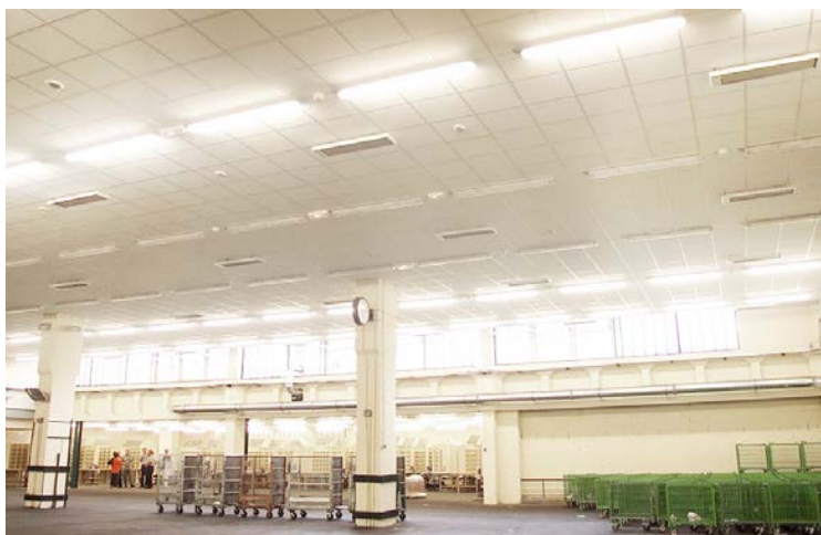
With radiant heaters, the heat is transferred to surfaces such as people, floors and fixtures. This creates comfort even in rooms with large volume.
