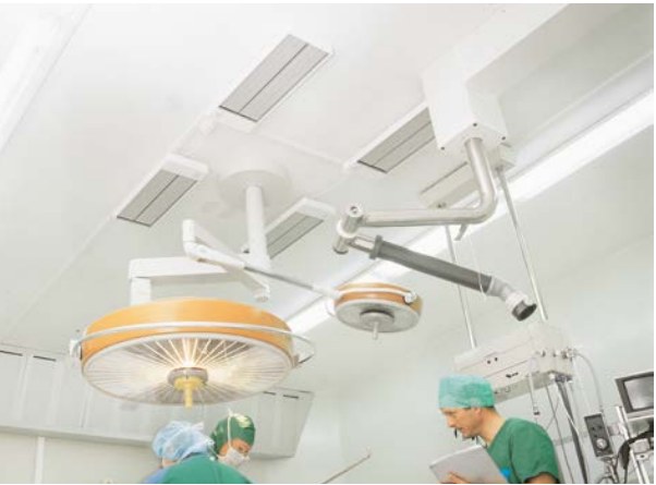
Heating with EZ200 is hygienic since it does not cause any air movements.
