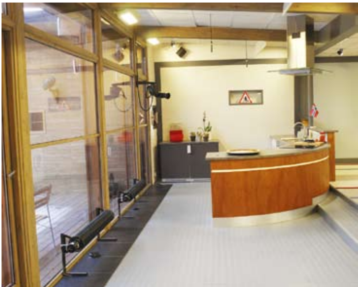
Installed by a window the ribbed pipe radiators effectively counteract cold draughts that frequently form by large glazed areas.
