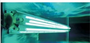
Installing parallel to the air-stream increases dwell time (contact time) with air
