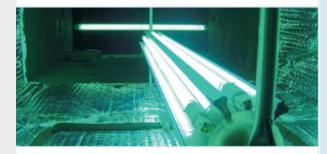
Severe chemical and odourapplications: a single Multi-split lamp working in conjunction with the UV bio-wall is installed up-stream
