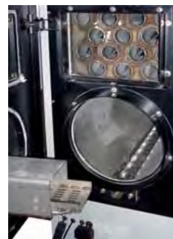
EXCHANGER AND COMBUSTION CHAMBER WITH A WORM GEAR TO REMOVE THE ASHES
