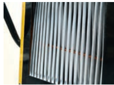
Wide spaces between evaporator tubes to prevent clogging
